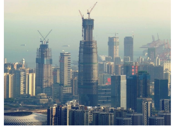
Shenzhen China Under Construction
